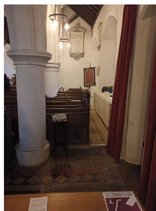
The South Aisle looking East
