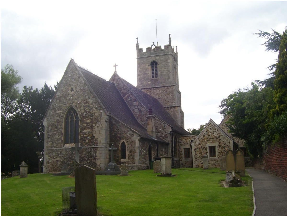
4 View from the East, with the Church Room addition on the right.
