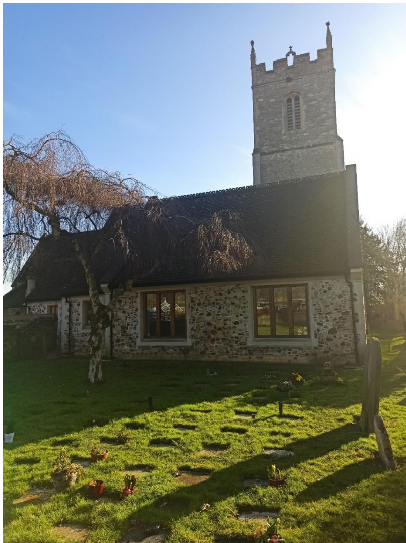
18 The exterior of the meeting room
