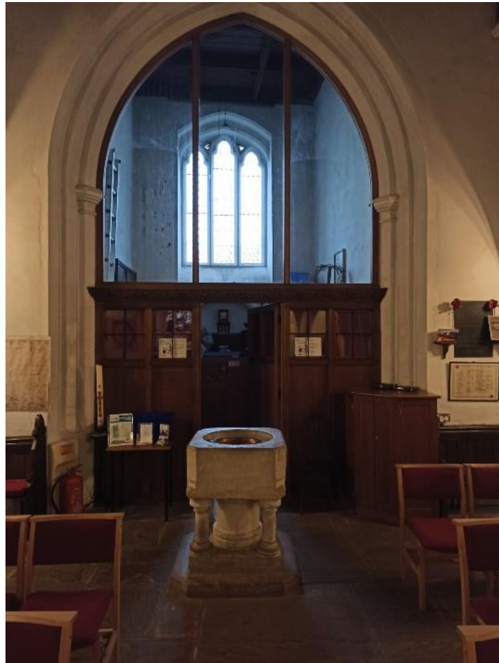
14 The nave looking West into the lower tower
