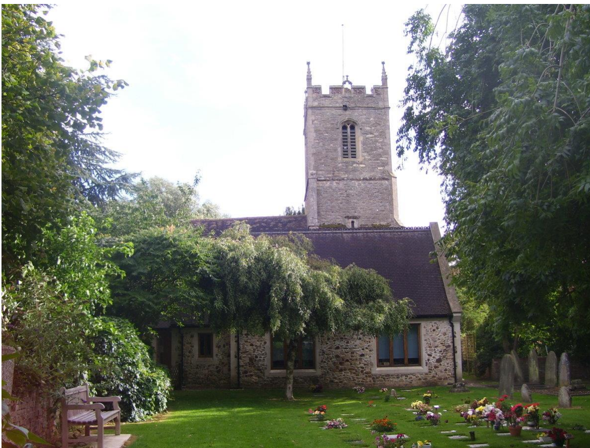
5 View of the North side showing the church room, from the cemetery.
